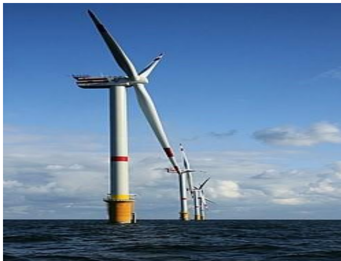
Figure 2-23 The general view of the offshore horizontal axis wind turbine
